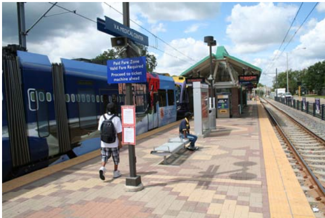
Light Rail at VA Medical Center, Minneapolis, MN
