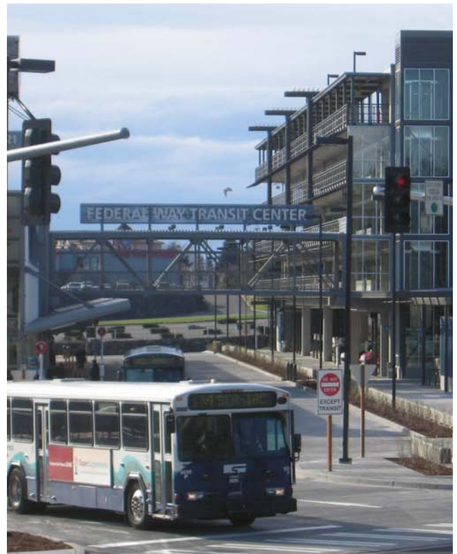
Integrating Park and Rides within transit centers improves journey options for passengers (Seattle, WA)
