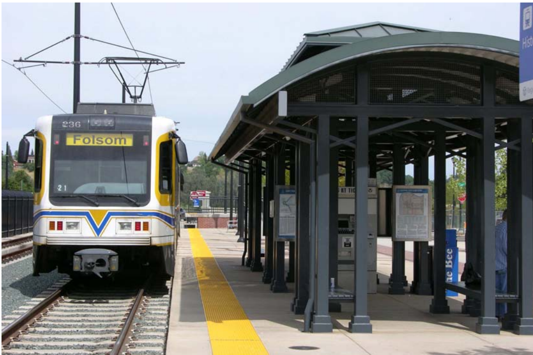
Light Rail extensions in the major corridors will connect more people to jobs and other major destinations.
