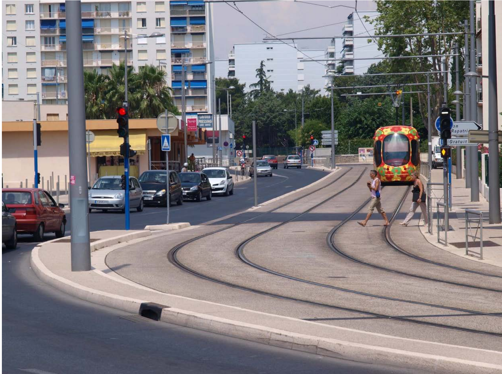
A complete street design with space prioritized for light rail (Montpellier, France).
