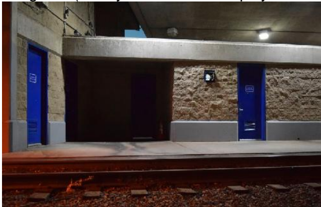
Image 24 (Poorly lit area near employee bathroom-nighttime)
