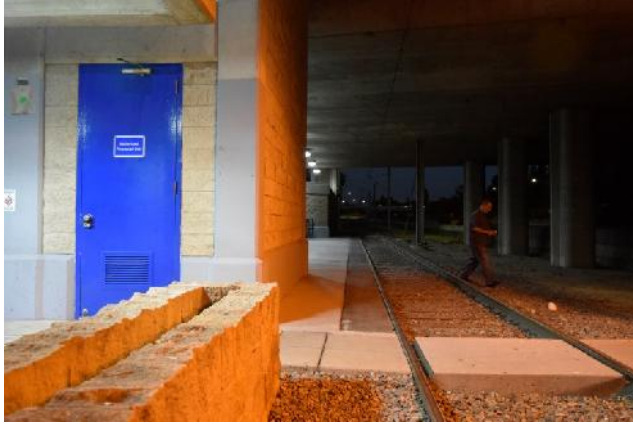
Image 23 (area to be posted with signage leading to employee bathroom)
