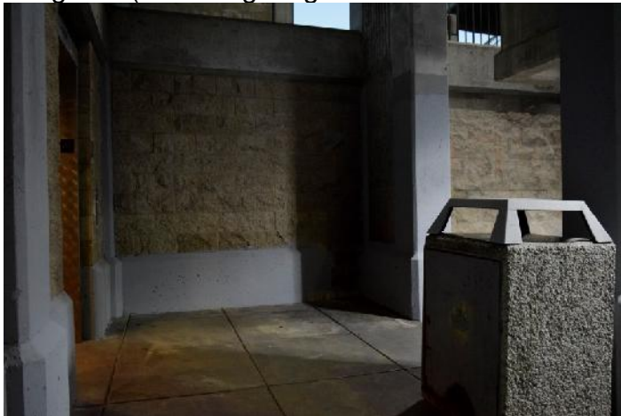
Image 15 (lack of lighting creates shadowed areas)
