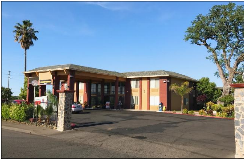
The Courtyard Inn (3425 Orange Grove Avenue), located a quarter mile from the Transit Center, will be redeveloped into an affordable housing complex.
